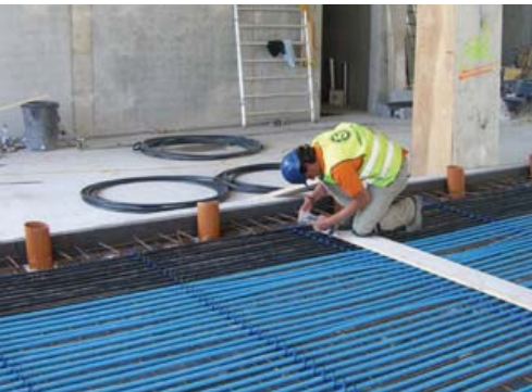
Installation Swedice rinksystem
